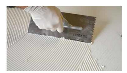
Mixing ratio:Component A: 92,6 parts by weight - Component B: 7,4 parts by weight. Mixture life:approx. 60 minutes.
